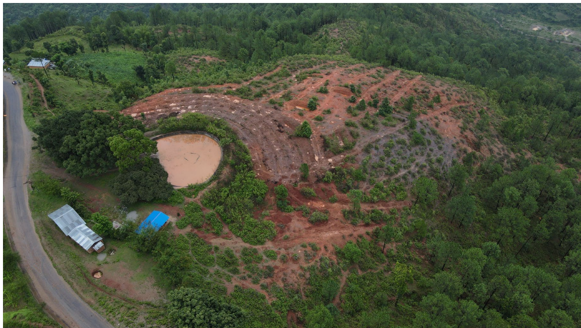
Photograph 12: Restoration of water recharge ponds and plantation in Ramecchap.
